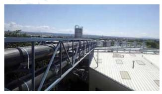
Cool Fit ABS Plus installed outdoors for the cooling unit of all the fermenting cellars at the Sierra Nevada Brewery.
