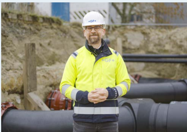
GF Piping Systems' Fabian Probe, Technical Manager for Infrastructure (Germany), was on-site, supporting the installation of GF's flow solutions, including GF's BIG couplers and MultiJoints.
