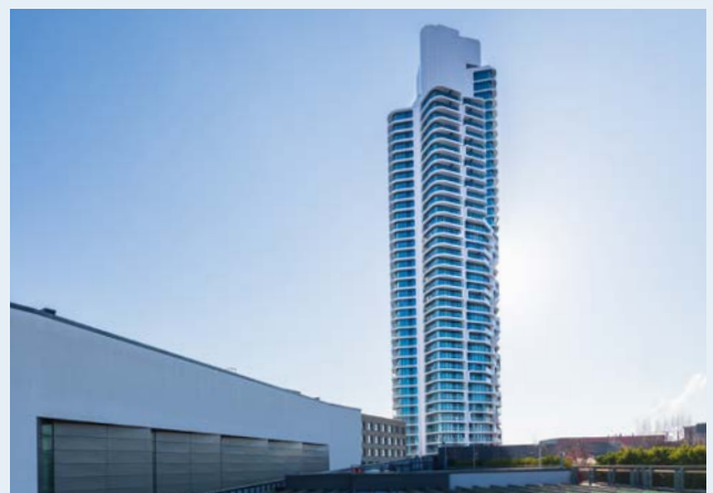
The Grand Tower in Frankfurt am Main, Germany's tallest residential building, features over 400 apartments equipped with GF Building Flow Solutions' heat interface units (HIUs) that meet the high demands of heating and cooling in these luxury homes.
