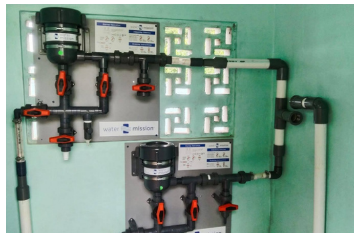
Two Erosion Chlorinators are part of the safe water solution for Oenoni.
