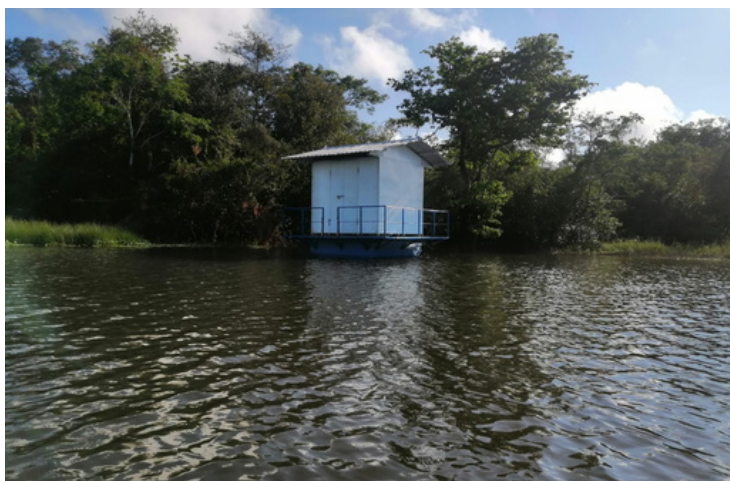
San Roque's floating pump station that was also built by staff and community members.
