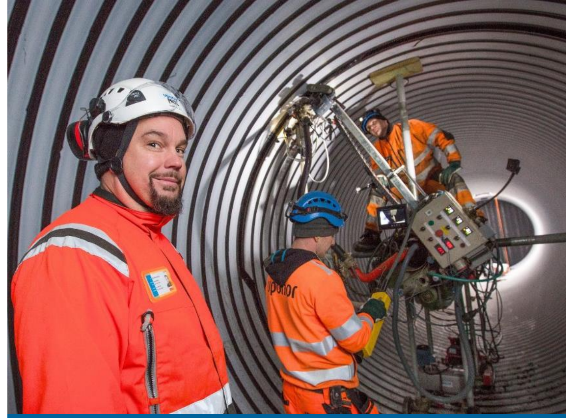
Prefabricated and integrated for efficient installation
